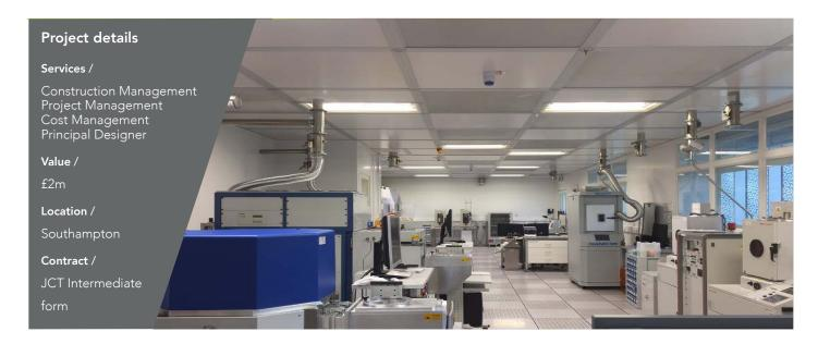
Management/coordination of multiple technically complex Long Term Maintenance/upgrade works within an extremely highly serviced research facility while the building remained operational. Works included chilled water system upgrade, replacement of Fan Filter Units, LED Lighting replacement and fibre drawer tower upgrade/alterations.
